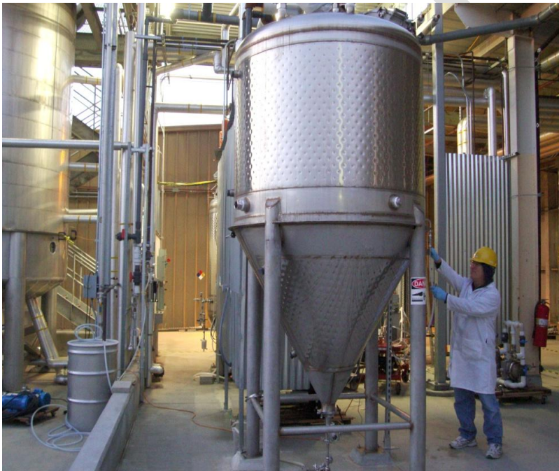
Employee checking biofuel tanks at Menom International in Rancho Bernardo
