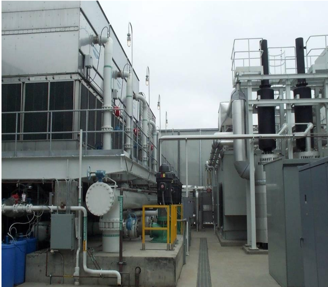
Johnson & Johnson's La Jolla R&D laboratory is cooled using reclaimed water
